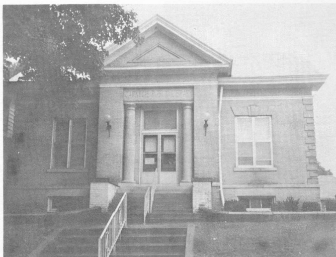
TOWN OF POSEYVILLE c.1900 Cale St. Poseyville
