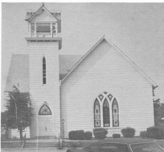
METHODIST CHURCH 1856 Many alterations after 1900 Lane Street Equality United Methodist Church
